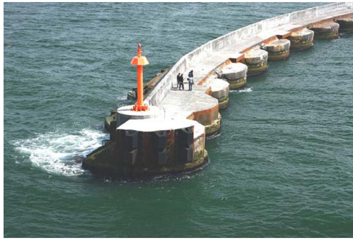
Photo 1.1: Hanstholm breakwater (Denmark). [8 - panoramio]
